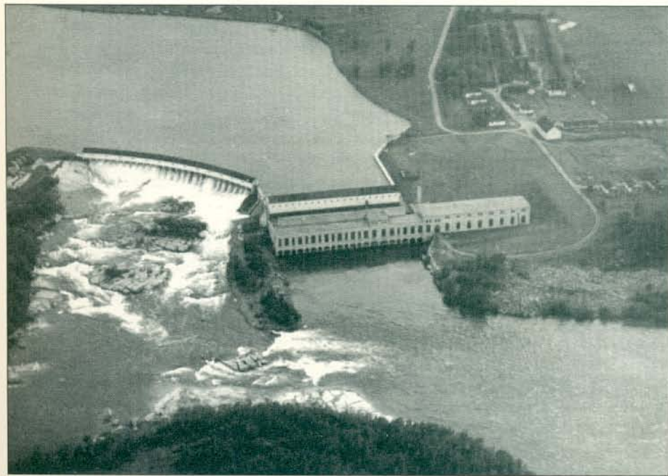
Pinawa Generating Station was located close to the Pinawa townsite, seen at upper right.
